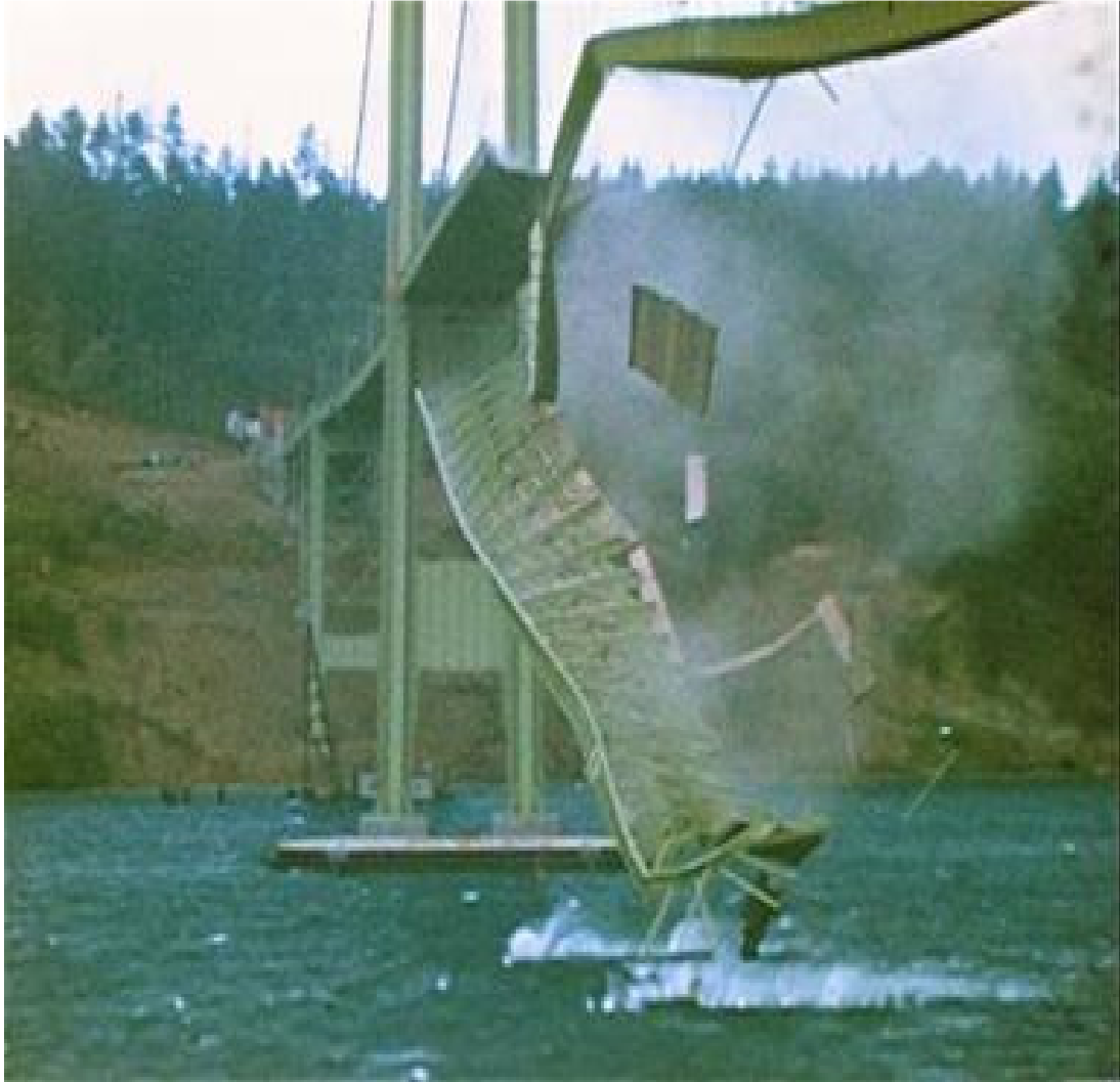
Figure 1-4- The destructive nature of VIV is best explained by the Tacoma Narrows Bridge Disaster in Tacoma, Washington, 1940
